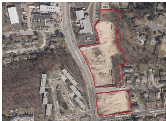
Aerial Photo of Site
